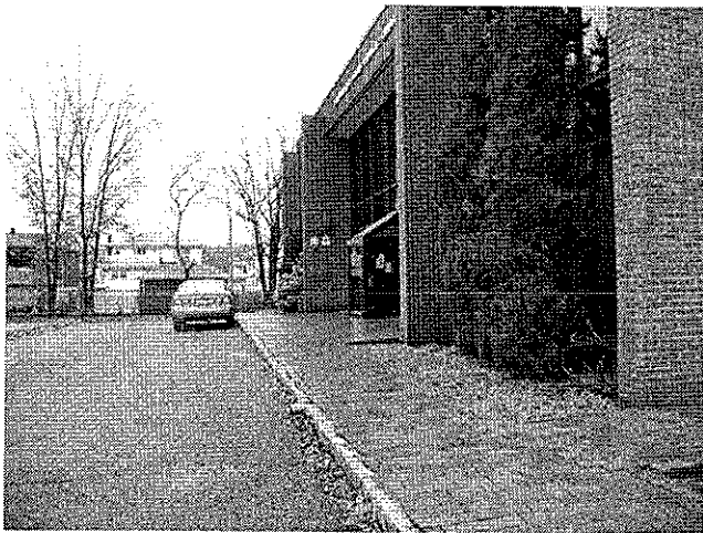
A23 _ Front Entrance
