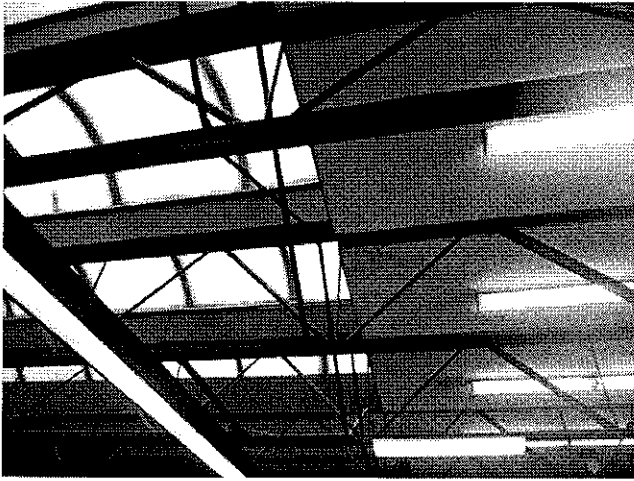
A25 _ Skylight and Ceiling Tile
