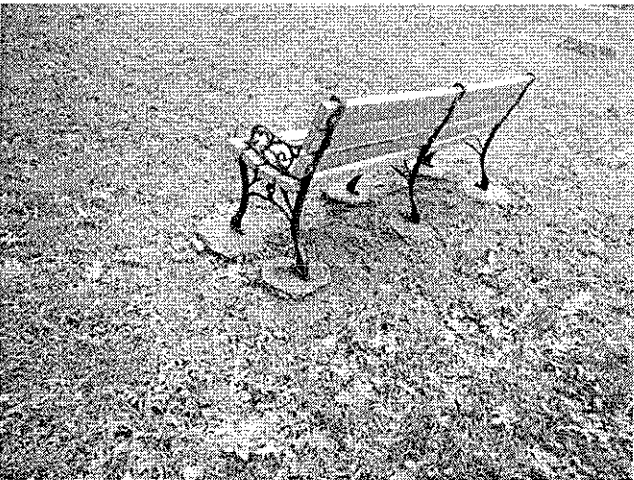
A11 _Exposed Footings
