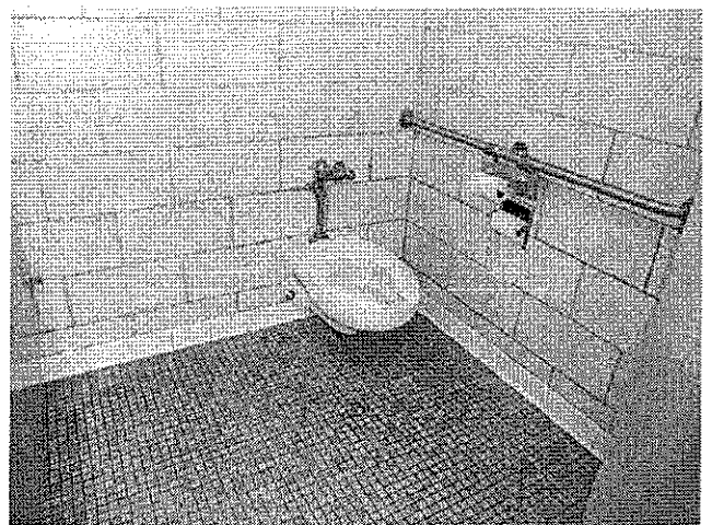
A18 _Men's Restroom
